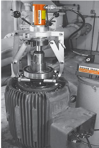
▶ Puller with a bearing pulling attachment was used to take a bearing off a utilities well pump motor.
