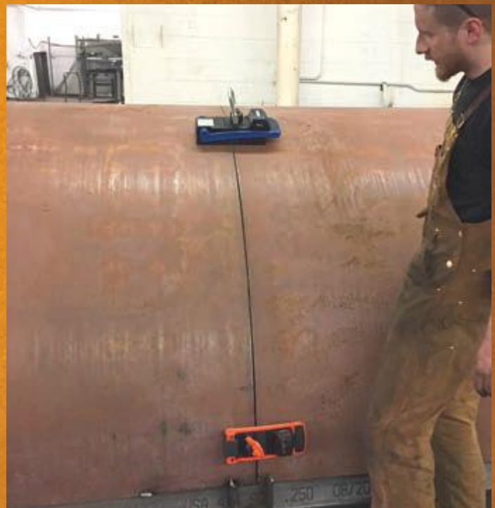
CONTAINER CONSTRUCTION—WROCŁAW/POLAND — MAREK
