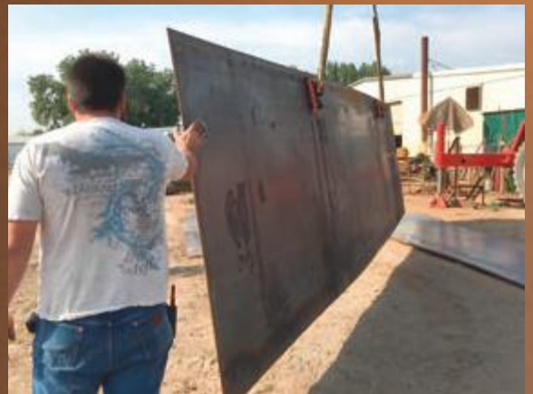
HALL CONSTRUCTION – BLOOMFIELD / USA – RICARDO
